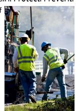
**WORK ZONE PROTECTIONS:** Various concrete, water, sand, collapsible barriers, crash cushions, and truck-mounted attenuators can help limit motorist intrusions into construction work zones.
